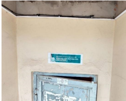
Fig. 7: Mounted misting nozzles at the entrance of the Robotics and Automation Laboratory
